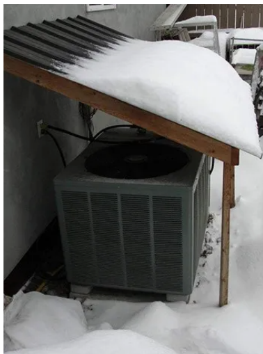
FIGURE 5 HEAT PUMP WITH ROOF
